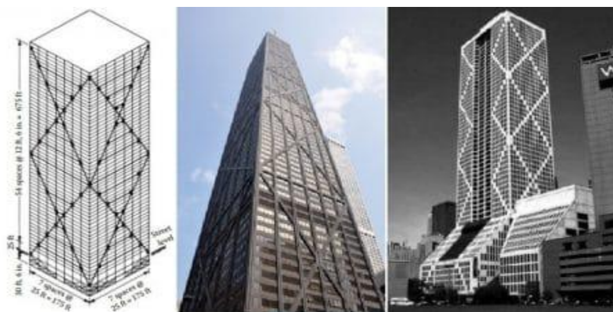
Figure 10. An example of a Braced-Tube Structures System ( https://ars.els-cdn.com )
