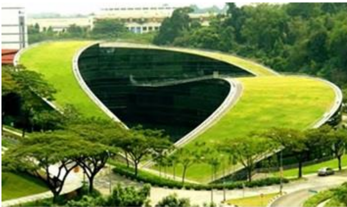
Fig 5. Green Roof URL:2
