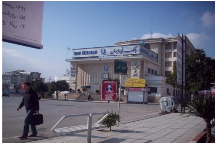
Figure 3: National Bank, after the addition of an extension building (Source: Writer)
