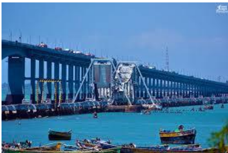
Plate 2. Pamban Rail Bridge near Rameswaram
