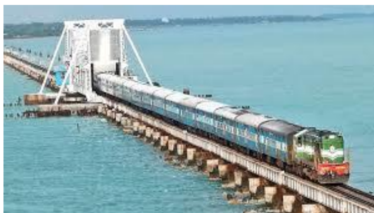
Plate 3. Train crossing Pamban Rail Bridge
