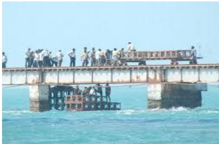
Plate 1. Pamban Rail bridge being repaired
