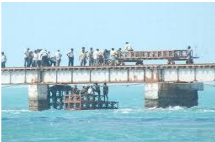
Plate 1. Pamban Rail bridge being repaired
