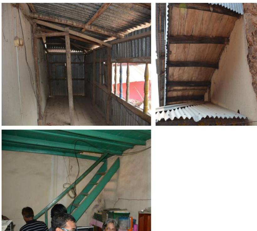
Figure 27-29: Above: cantilever verandah interior view and its construction system,
