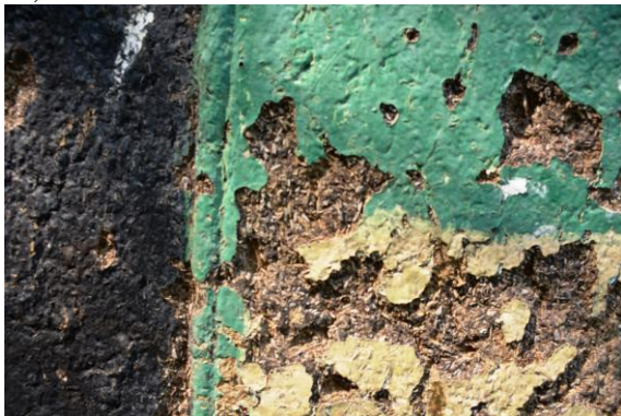
Figure 20: The different layers of bitumen, rice husk and paint over mud blocks of case study 4
