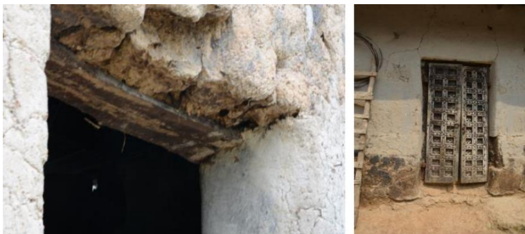
Figure 25-26: Left: palm plank for lintel at case study 2 and wooden frieze at case study 3
