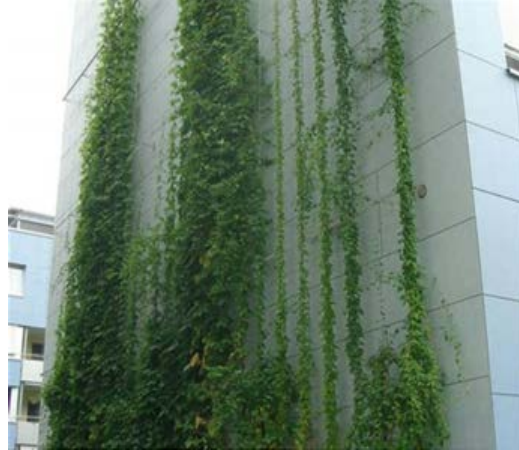
Figure 4. Green View Cable System (Source: atlantiscorporation.com)
