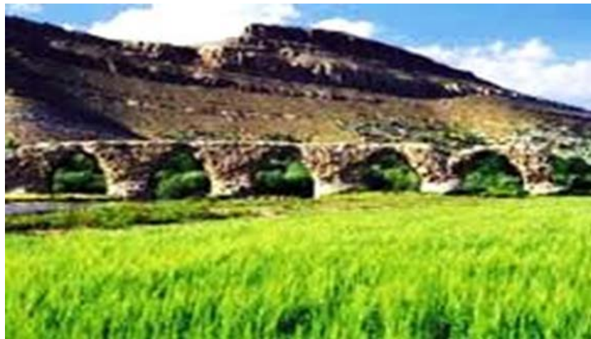
Figure 3: Picture of the ruins of the Shapour khast bridge
