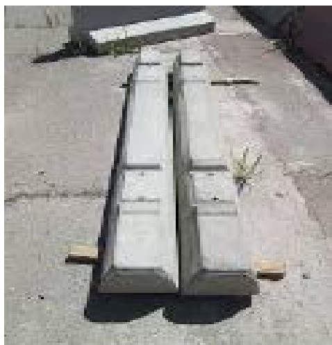
Figure 1. The pre-stressed sleeper B 70
