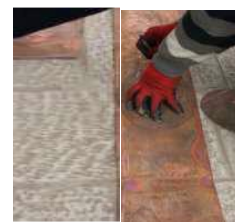
Image 10: Surfacing, measuring on copper sheet
