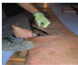
Image 11: Surfacing, cutting copper sheet
