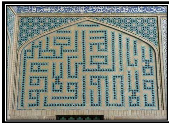
Figure 5: The Moaqali brick work (Source: www.beytoote.com )
