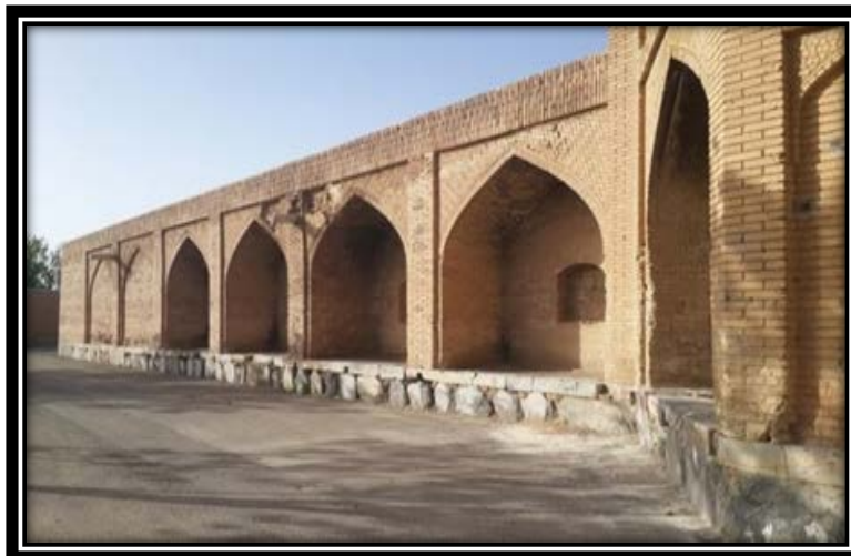
Figure 6: The caravanserai of Shah Abbasi Sheikh Ali Khan in Isfahan (source: authors)
